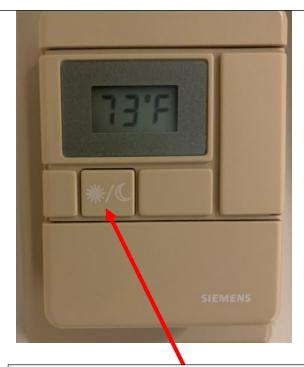
Pushing this button in for 1 full second will give your room 4 hours of occupied time. After 4 hours, push again if you continue to be in your room. **NOTE:** Subsequent pushes of the button will not shut off the unit nor add hours. It will however start the 4-hour time over again. (Example: Pushing at 8 AM, it should go till noon, pushing again at 10 AM will have the unit shutting off at 2 PM.)
