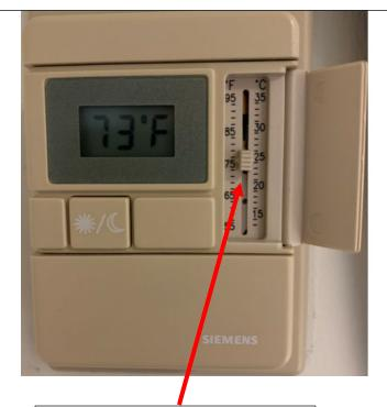
You also have some level of control by adjusting this slide. You can adjust between 75 and 82 degrees. This thermostat only works for cooling.
